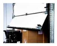
Double Knockout Header Allows the door to knock out in both directions at the top of the door opening. (vertical lift track only)
