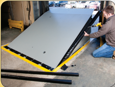
ENERGY GUARD® Retrofit Kit Installation
